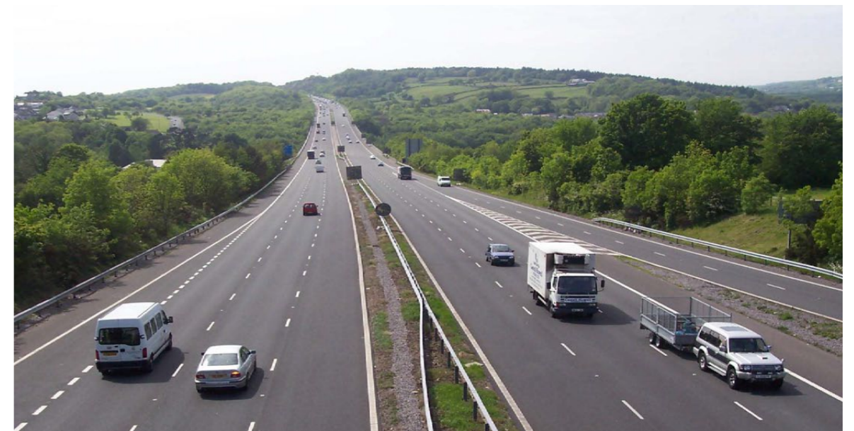
View of the M4
