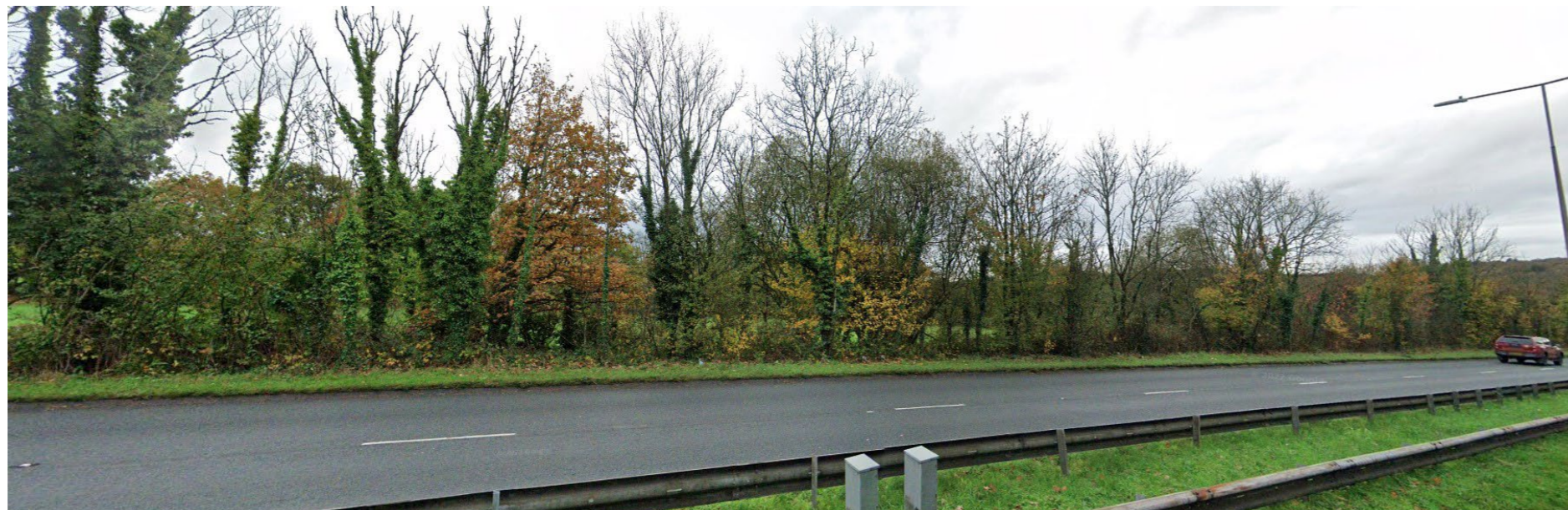
View of the site boundary from the A4063
