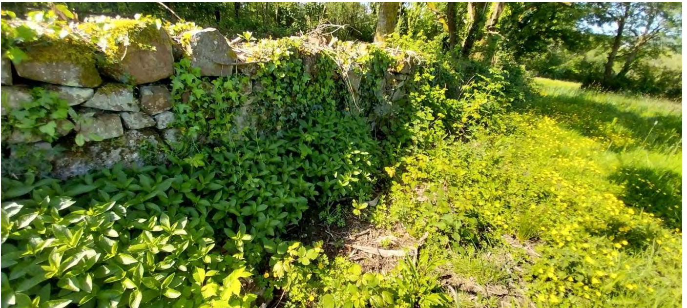
Photo: Historic stone wall (TN6.0) along southern boundary of southern section of woodland. Note presence of Dog Mercury Mercurialis perennis at base of wall indicating ancient woodland origins for the remainder of the site, not currently forming part of the 20212 AWI.
