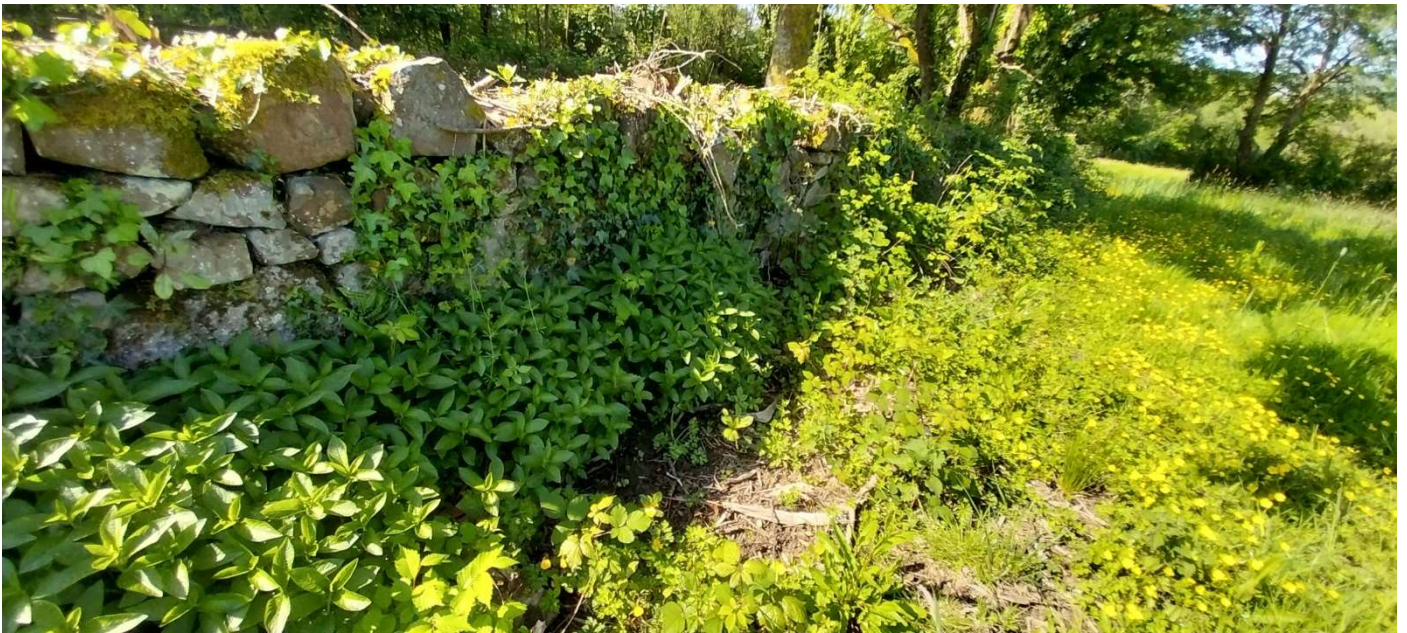
Photo: Historic stone wall (TN6.0) along southern boundary of southern section of woodland. Note presence of Dog Mercury Mercurialis perennis at base of wall indicating ancient woodland origins for the remainder of the site, not currently forming part of the 20212 AWI.
